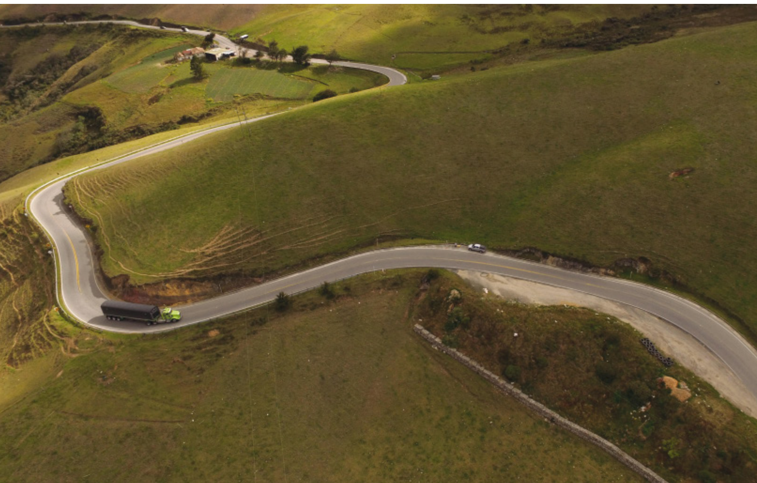
Roadway and bridge inspection services
