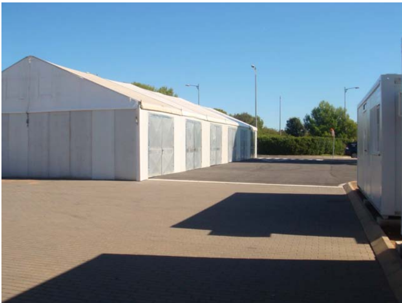
Vehicle preparation area and office area, external view
