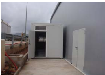
Office area, external view (KD3)
