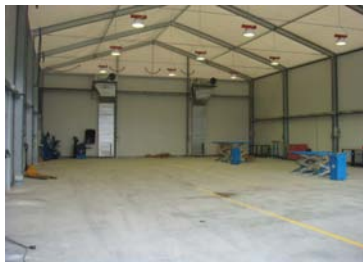
Vehicle preparation area, internal view (KD1, KD2, KD3)
