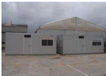
Office area, external view (KD1, KD2)
